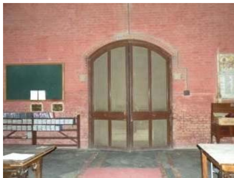
Figure 5 Inside view at the West Entrance, Lahore Cathedral. (2014)
