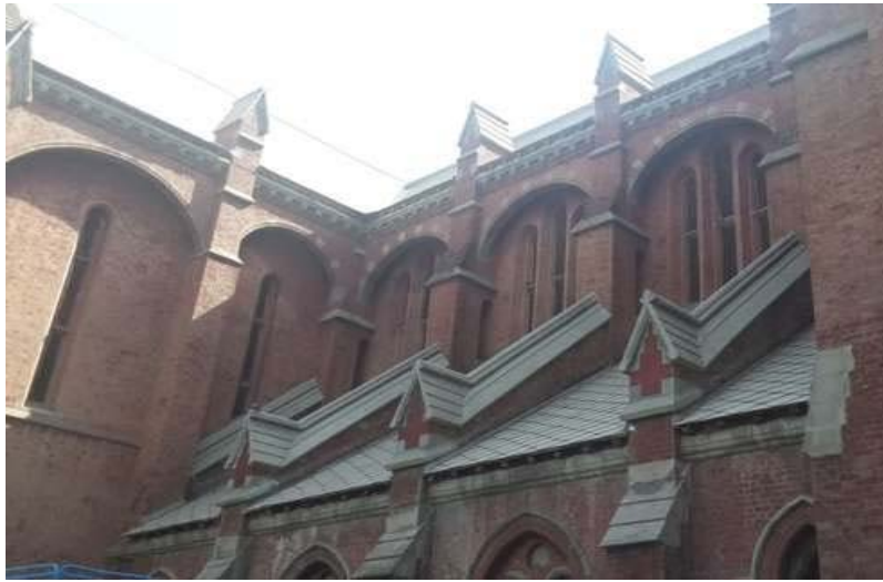
Figure 12 External view of the Central Vessel Window at Cathedral, Lahore
