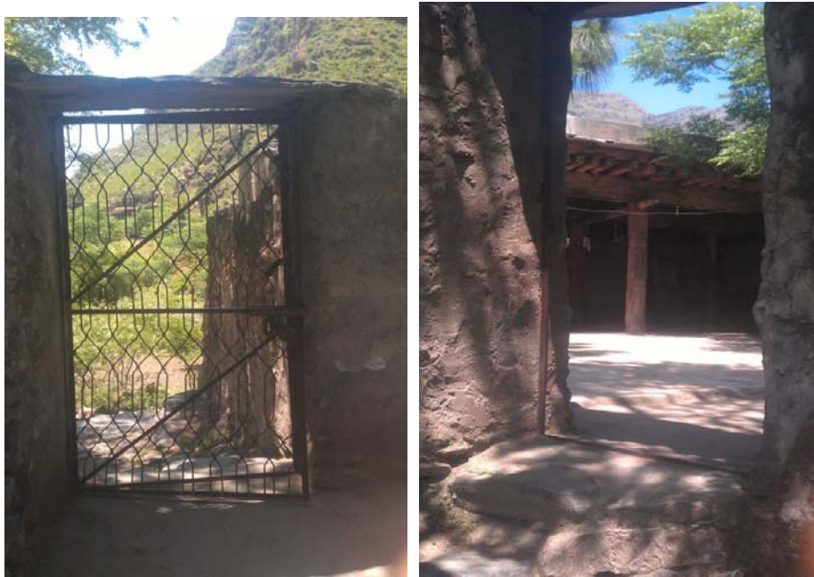
Figure 1: Main entrance viewed from inside (left) and outside (right), showing the iron-grilled gate and cemented boundary walls; the dry riverbed is visible at the base of the approach
