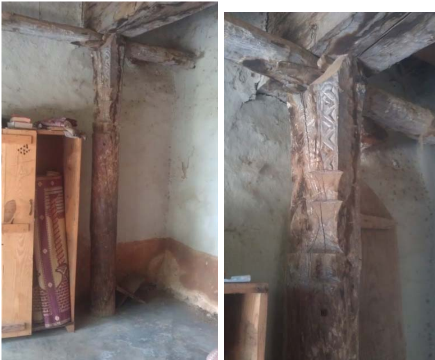
Figure 9: Third pillar of the 1st row: lime-plastered surface with only traces of zig-zag incised lines surviving at the shaft head
