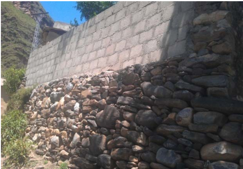
Figure 4: Outer view of the boundary walls showing stone steps compensating for the sloping hillside terrain
