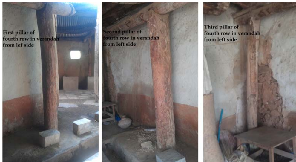
Figure 14: All three pillars of the fourth row of the veranda, added in 2000: plain, undecorated round shafts standing in stark contrast to the carved columns of the first row immediately adjacent
