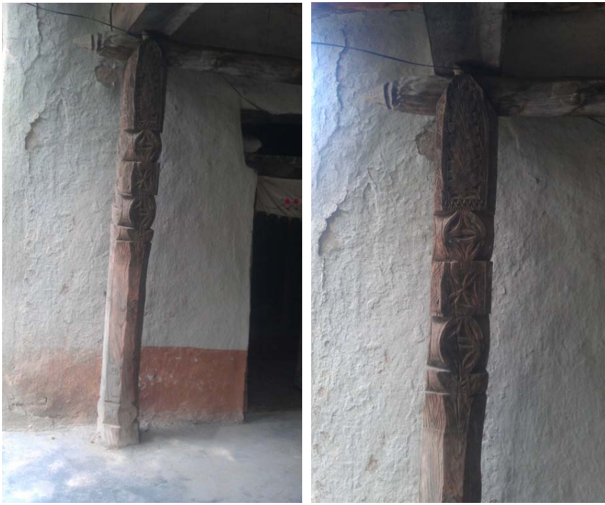
Figure 6: First pillar of the 1st row: front face (left) and northern face (right) showing carved rosette flowers, leaf garlands, and four-petalled medallion, the most complete surviving decorated surface in the mosque
