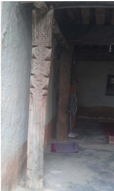
Figure 7: Northern face detail of the 1st pillar, 1st row, showing the differentiated decorative programme applied to the upper shaft, evidence of the craftsman's attention to multi-face composition
