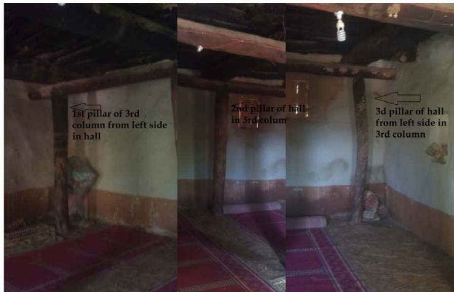
Figure 17: Third column of hall pillars: round shafts donated in 1998, showing fire-blackening from prior domestic use as kitchen structural columns
