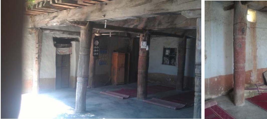
Figure 12: Third pillar of the second row of the veranda (two views), showing round section and zig-zag incised ornament
