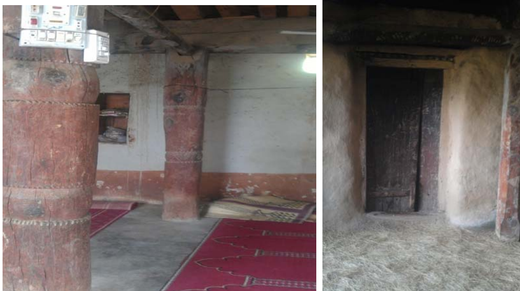
Figure 24: Floor surfaces of the prayer hall: original irregular stone-and-earth floor surviving in limited areas (left); modern machine-cut stone replacement introduced in successive repairs (right)
