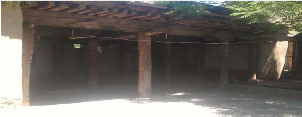
Figure 3: Eastern and southern walls viewed from the veranda, showing mud-plastered stone construction with stucco border finish
