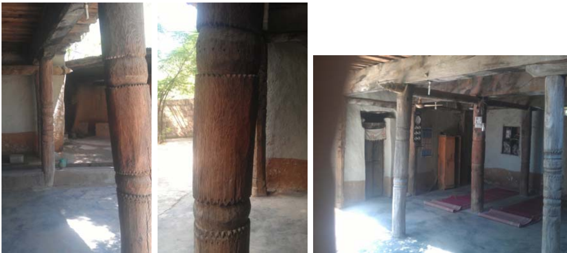
Figure 10: First pillar of the second row (three views): round section shaft with zig-zag and circle incised decoration, transferred from Dewana Baba mosque c.1975
