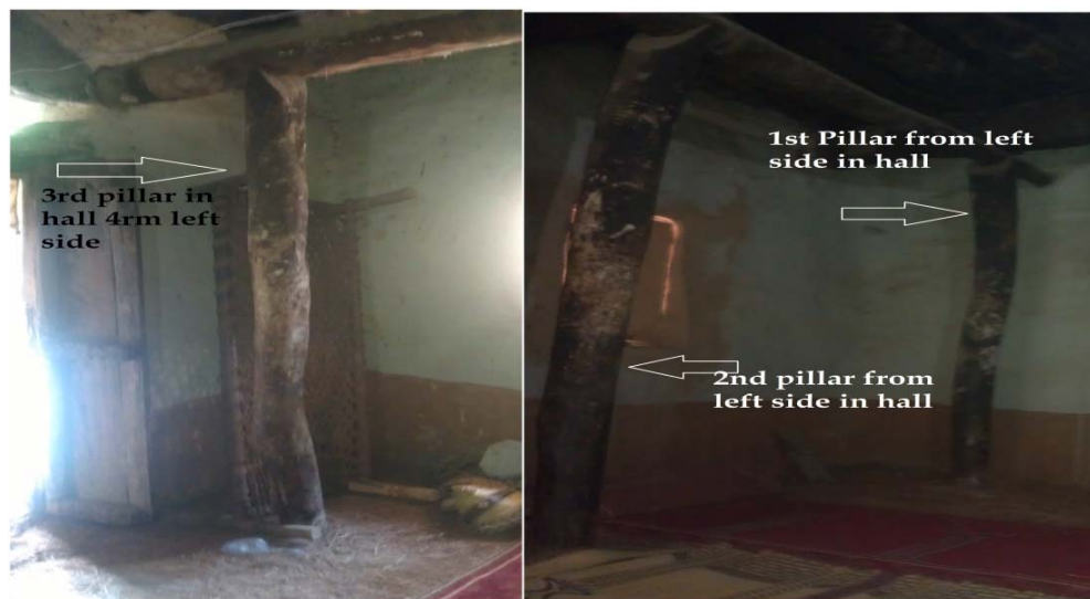
Figure 15: All pillars of the first column in the prayer hall: round, undecorated shafts from Dewana Baba mosque, installed 1975
