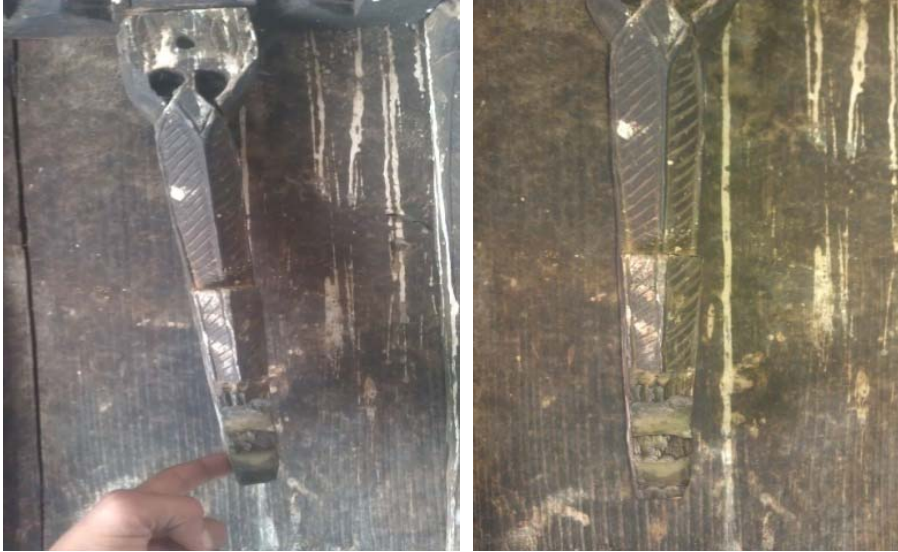
Figure 21: The indigenous wooden locking mechanism on the right door frame: dart-and-slot fixing with leaf-and-line carved ornament, a rare in-situ survival of a vanishing craft tradition
