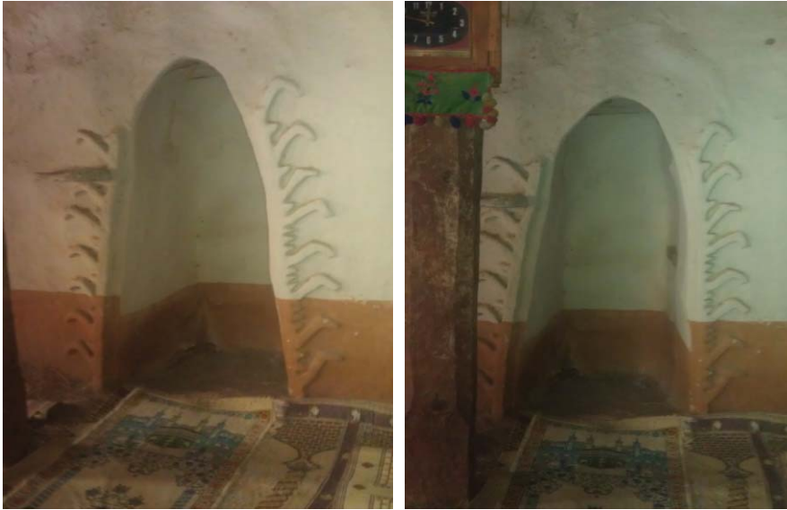
Figure 18: The mihrab in the prayer hall western wall: mud construction with raised-relief ornament applied by community women in 2000 (left, right), and stone candle ledge
