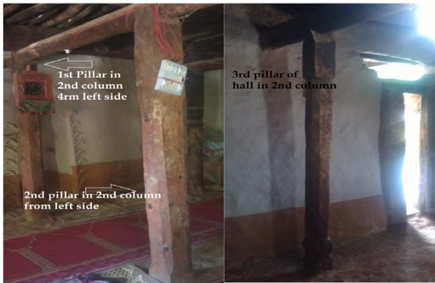
Figure 16: Second column of hall pillars: rectangular-section elements added in 2000, showing less accomplished workmanship reflecting the loss of specialist craft skills
