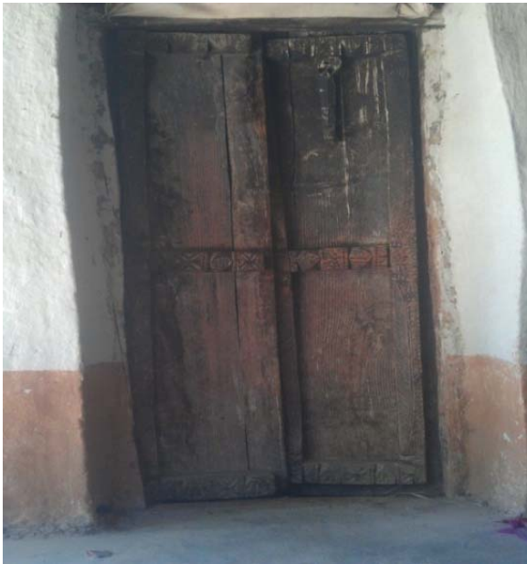
Figure 19: The main door of the prayer hall: double-leaf construction in ranzra hardwood, the oldest surviving joinery element of the mosque
