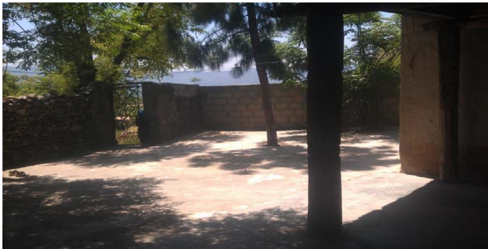
Figure 2: Eastern and northern walls showing the junction between original stone-and-mud fabric (right) and later concrete block reconstruction (left)
