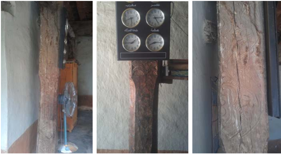
Figure 8: Second pillar of the 1st row: front face with clock fixture obscuring carved surface (left); northern face showing traces of branching flower motif (centre, right), the clock represents an entirely reversible but as yet unreversed loss
