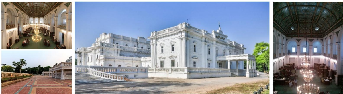
Figure 5: Architectural Features of Montgomery Hall (Source: Government of Punjab, n.d. )
