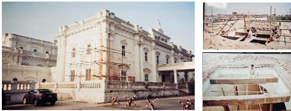
Figure 6: Renovation of Hall In 2012 (Source: PWD Department)
